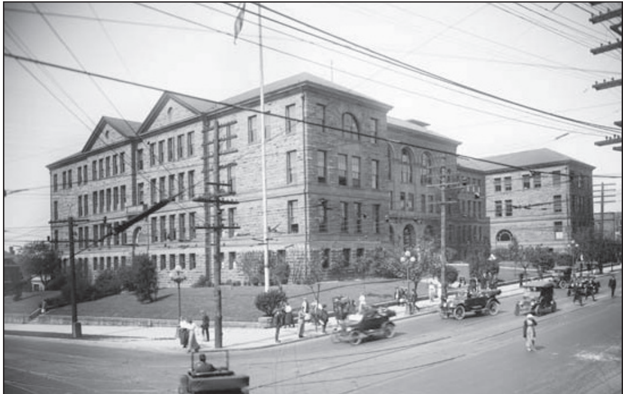
Figure 6 • Central High School/Broadway High School (W.E. Boone & J.M. Corner, 1902)
