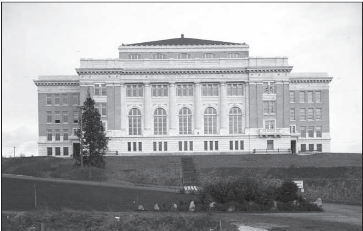
Figure 12 • Franklin High School (Edgar Blair, 1912, City of Seattle Landmark)
