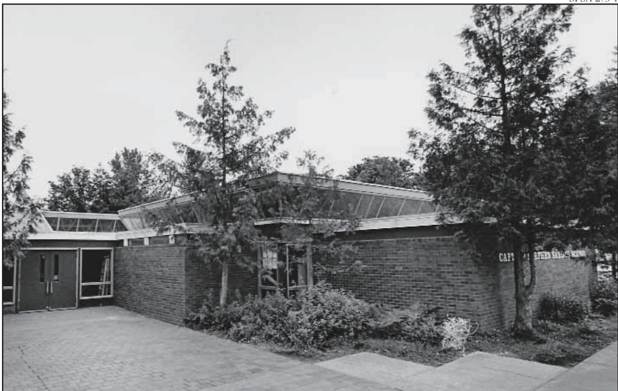
Figure 20 • Captain Steven E. Sanislo School (Sullam, Smith & Associates, 1970)
